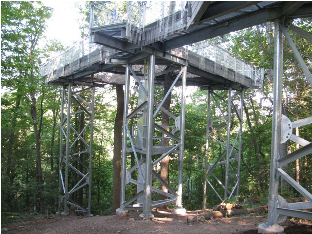
Photo 4: Steel towers supporting framing around trees and cargo netting
