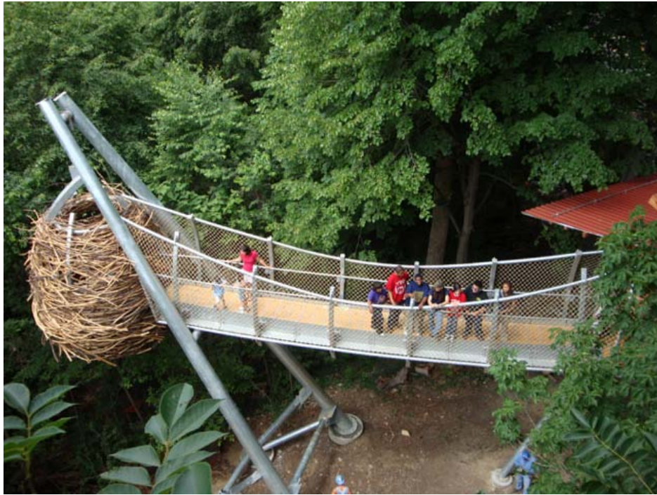
Photo 3: Glulam "Bridge" & steel "Birds Nest" with steel monopoles & micropile foundations
